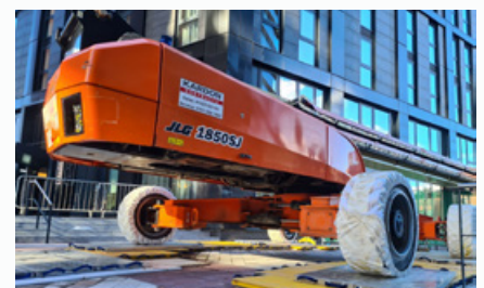
POWERED ACCESS SET UP
